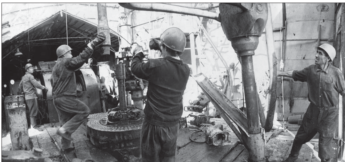
Drilling of the oil well led by M. Grin's best brigade. Aznakaevo drilling department of the 'Tatneft' association. Almetyevsk. 1975. National Archive of the Republic of Tatarstan
