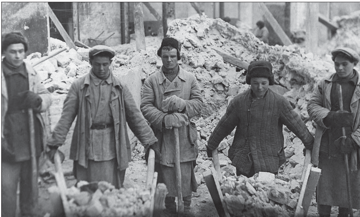
Members of the shock brigade of bricklayers at the construction of the Kuybyshev Kazan Chemical Plant. Kazan. 1930s. State Archive of the Historical and Political Documentation of the Republic of Tatarstan
