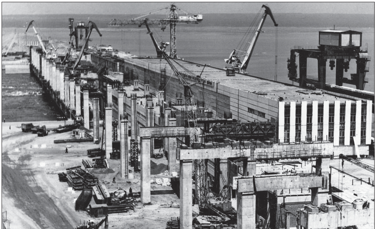
Nizhnekamsk hydro-electric power station. Nizhnekamsk. 1980. State Archive of the Historical and Political Documentation of the Republic of Tatarstan
